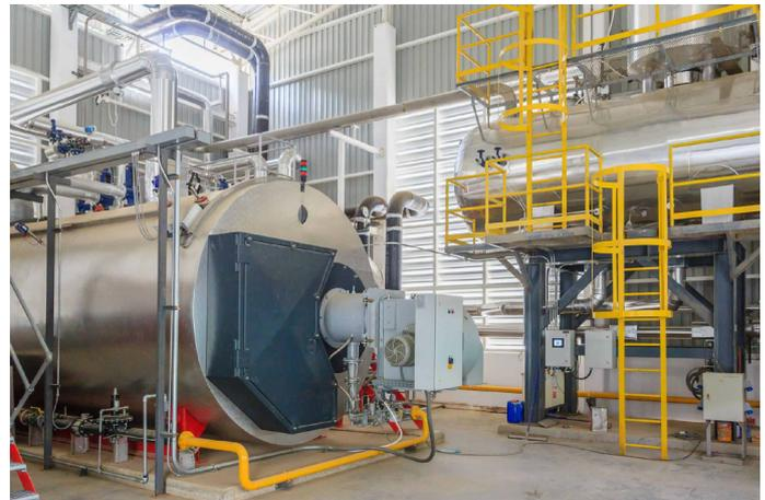
Individual physical parameters are combined within the monitoring system analysis process to provide calculated and computed datapoints such as heat flow and boiler efficiency level.
